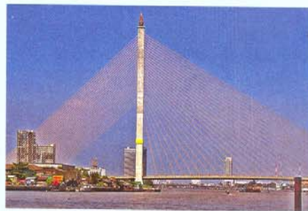
Figure 1.116 Rama 8 Bridge, Bangkok, Thailand
