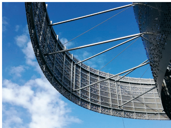
Fig. 5 Construction of the upper windings with frames and generatrices.
