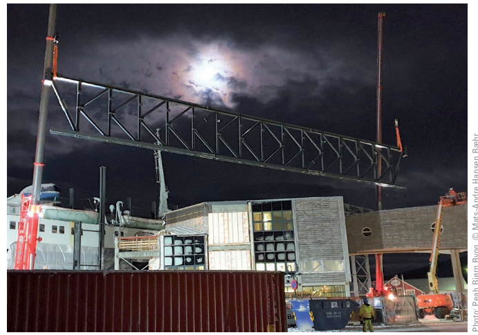
Fig. 10 Installation of truss over the Triangular Building
