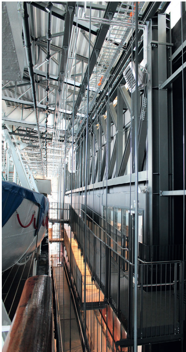
Fig. 9 Visitors can enter the ship from suspension ramp hanging in tension cables from the roof trusses
