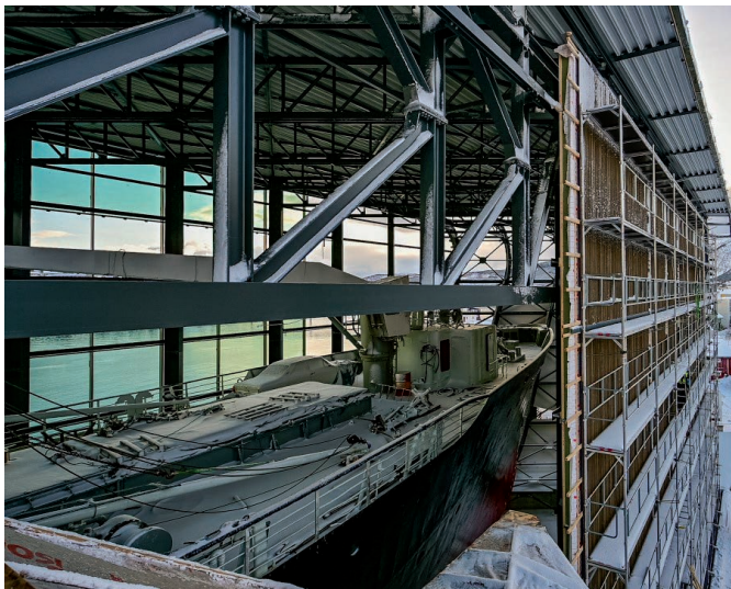
Fig. 6 The large truss in the Protective Building designed for deflection over the Triangular Building
