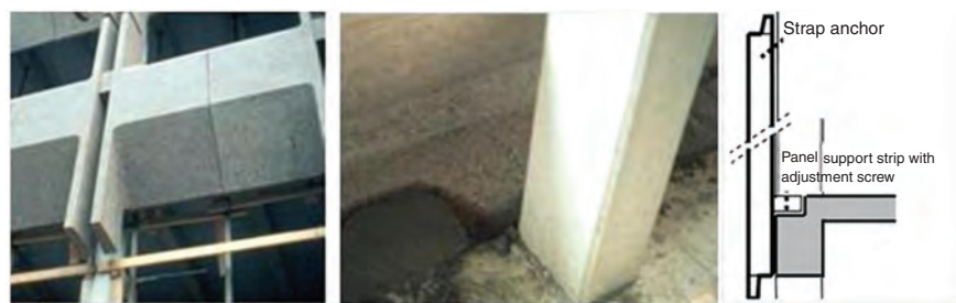
Figure 11.3 Non-load-bearing panels, mounting.
