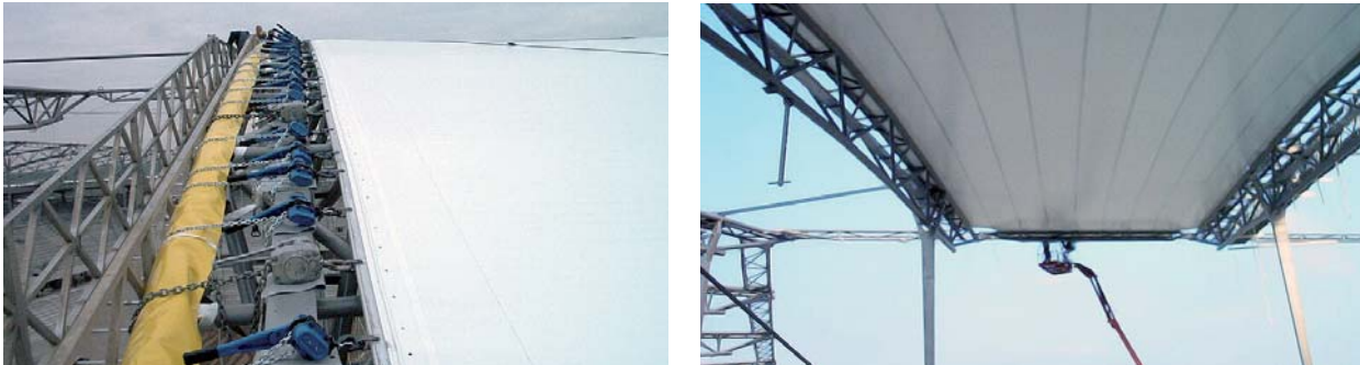
Fig. 100: Pulling in and tensioning the membrane for the stand roofing at stadium Volkswagen Arena Wolfsburg, Germany
