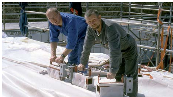
Fig. 118: left: Repair work with a hot air pistol; right: Welding of partial surfaces of Glass/PTFE membrane at the Munich Waste Management Office (AWM), Germany
