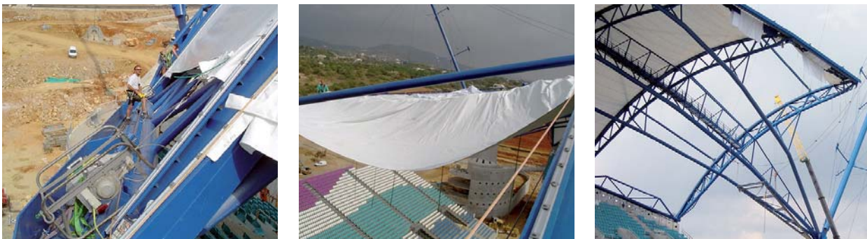
Fig. 101: Pulling in and tensioning the membrane for the stand roofing at Estádio Intermunicipal Faro, Portugal
