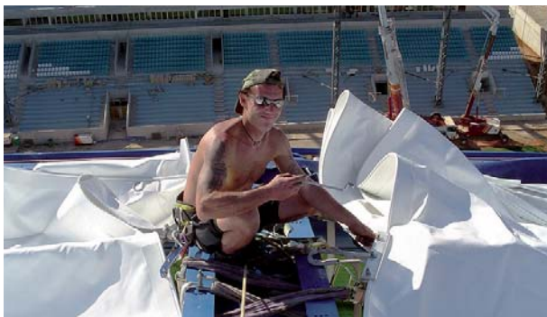
Fig. 104: Tensioning of high point surfaces with different strip layouts
