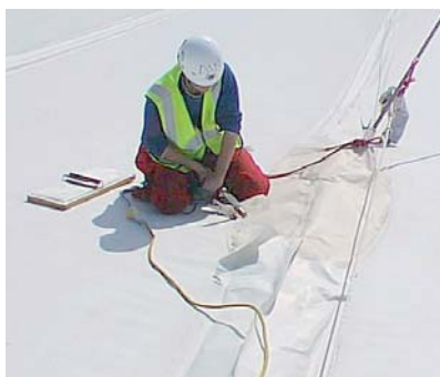
Fig. 118: left: Repair work with a hot air pistol; right: Welding of partial surfaces of Glass/PTFE membrane at the Munich Waste Management Office (AWM), Germany
