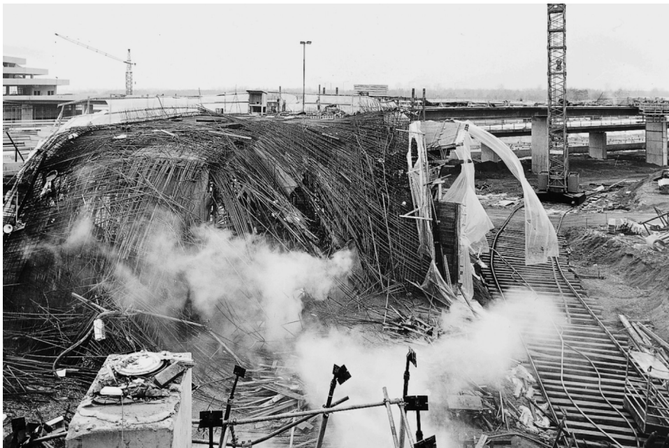
Fig. 11.1 Collapse of supporting scaffolding for a bridge ramp at Cologne-Wahn airport. 1995, Case 11.45
