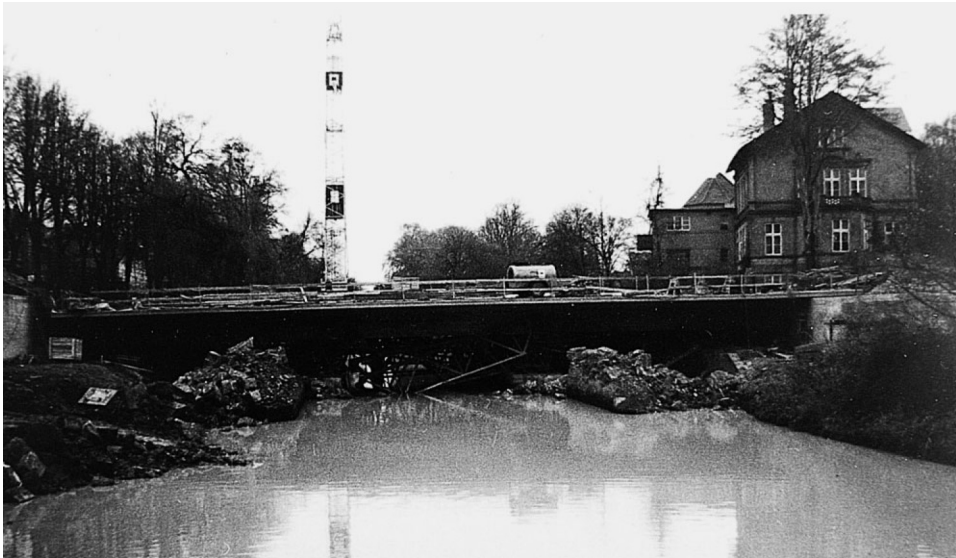
Fig. 11.8 Scaffolding collapses caused by settling of temporary foundations
