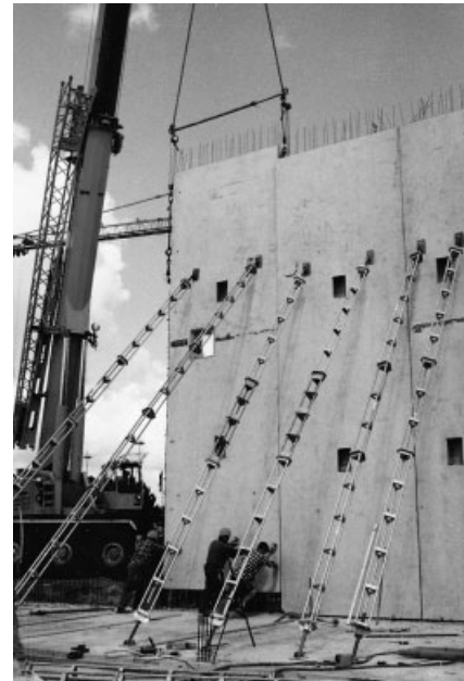
Fig. 2.92 Use of composite precast/in situ concrete wall for tall walls (SysproPART system)
