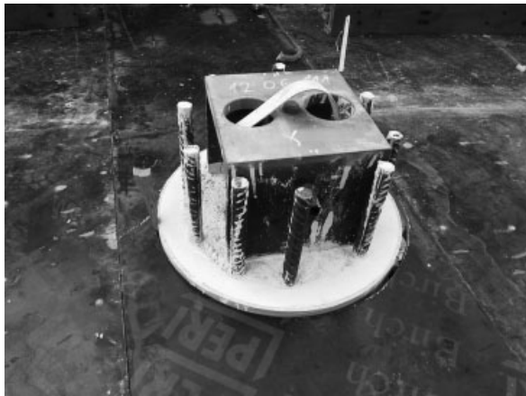
Fig. 2.90 Butt joint between precast concrete columns for Triangel Tower in Cologne (contractor: Züblin)
