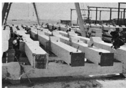
Fig. 2.96 Precast concrete column complete with precast concrete foundation (contractor: Bachl)
