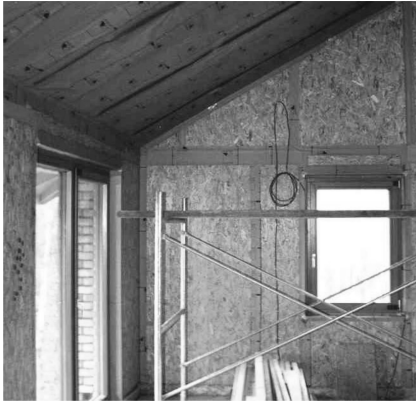
Figure 1.4. Taped OSB as air barrier.
