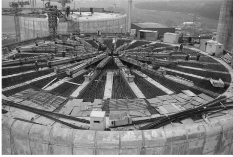
Fig. 4.5 Gundremmingen B and C reactor building roof structure, with precast wedge-shaped laid precast segments with cast concrete added locally [17]
