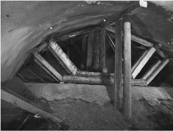
Figure 2-2 Timbering as emergency support after a collapse in the Euerwang Nord Tunnel [136]
