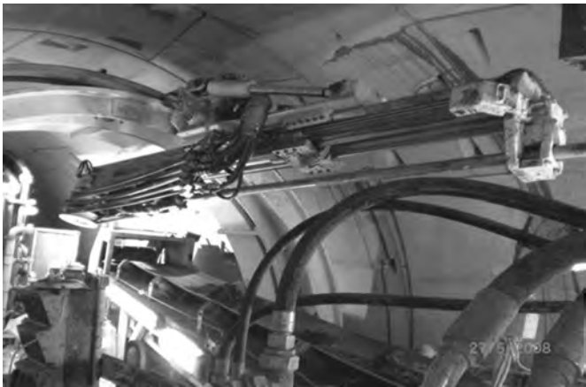
Figure 14.5 Probe drilling equipment used in the Melen project.
