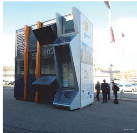
Figure 1-1 A mobile façade mock-up prepared by the coordinator of the project Züblin AG, will demonstrate in real-scale innovative BIPV glass-based technologies for the building envelope developed in Construct PV. The mockup, originated by the collaboration of Züblin with UN Studio, Fraunhofer ISE and Meyer Burger, demonstrates variants and possibilities in terms of architectural and technological design/manufacturing of BIPV systems for the building skin, showing different façade systems for glazed BIPV modules. It will be exhibited around Europe in the next years so that it will become a mobile demonstrative facility (more information at www.constructpv.eu ).
