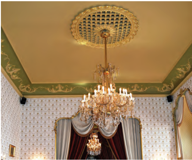
Figure 7.4 Example of a chandelier suspended from just one fixing point (photo: Scheller).
