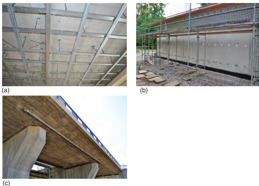
Figure 7.7 Real examples of multiple fastenings for non-structural systems: (a) fastening a support framework for a suspended ceiling (photo: Scheller), (b) fixing points for attaching continuous vertical members for a façade support structure (photo: Küenzlen), (c) fastenings for a pipe (photo: Küenzlen).
