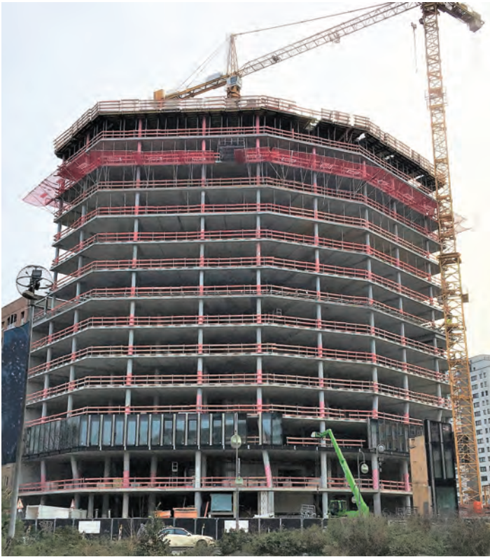
Figure 4.10 Example of the construction of a high-rise building: Fitting-out work (e.g. services and façade cladding) is already in progress on the lower floors while the upper floors are still being concreted (photo: Scheller).
