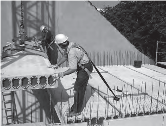
Figure 4.2 Positioning a prestressed hollow-core slab unit.
