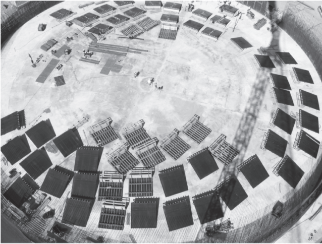
Fig. 8.10 Preparing the wall formwork elements.
