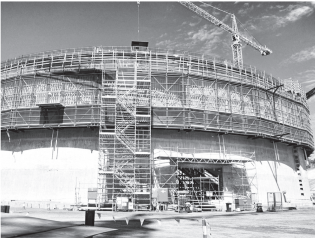
Fig. 8.8 Temporary opening.
