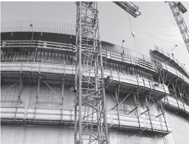
Fig. 8.11 Climbing formwork being repositioned for next lift.
