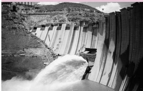
The cover picture shows the Kaste dam in Lesotho 1996 during construction. Due to high rainfall in the beginning of 1996 the control outlet had to be opened to limit the increase of the water level. The 1996/97 finished dam has a length of 710 m and a height of 185 m. The dam is part of the Lesotho Highlands Water Project which includes several dams and was planned to ensure water supply to major industrial centres of South Africa.
